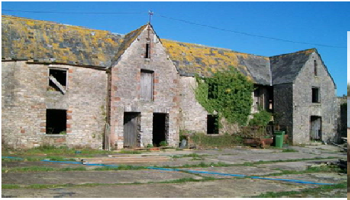
Churston Court Barns: This development, completed in 2014/15, shows how sensitive redevelopment can bring new life to old buildings.
